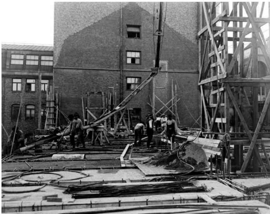
Building site in Stockholm around 1900.
